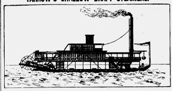
STEAMERS have been found by experience to be the best type of vessel for shallow river navigation desers. Yankow have constructed a large number of successful examples for all parts of the world. It is system are constructed when required, to draw as little as 6 inches. We have the sternwheelers "Mosquito" and "Herald" for the British Government, for servi
