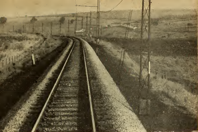
Electrified section of the Paulista Railway
