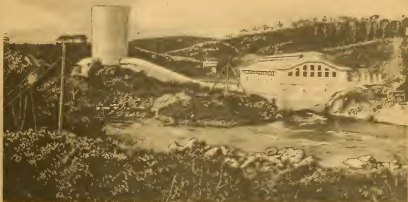
USINA HYDRO-ELECTRICA — BANANEIRAS, BAHIA
