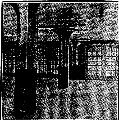
CONSTRUCTIONS IN REINFORCED CONCRETE Speciality - FLAT SLAB SYSTEM. Ford Building - São Paulo - built by us is the first example of this system in Brazil.
