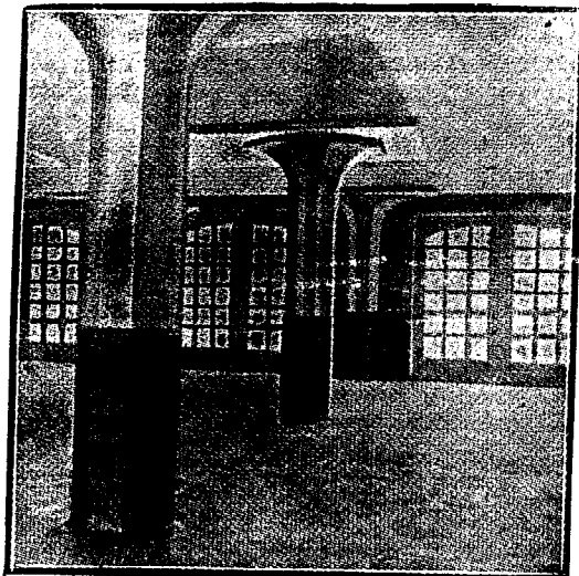
CONSTRUCTIONS IN REINFORCED CONCRETE Specialty - FLAT SLAB SYSTEM. Ford Building - São Paulo - built by us is the first example of this system in Brazil.
