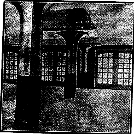
CONSTRUCTIONS IN REINFORCED CONCRETE Speciality - FLAT SLAB SYSTEM. Ford Building - São Paulo - built by us is the first example of this system in Brazil.
