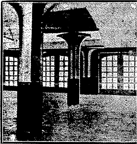
CONSTRUCTIONS IN REINFORCED CONCRETE Specialty - FLAT SLAB SYSTEM. Ford Building - São Paulo - built by us is the first example of this system in Brazil.
