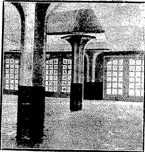
CONSTRUCTIONS IN REINFORCED CONCRETE Speciality - FLAT SLAB SYSTEM. Ford Building - São Paulo - built by us is the first example of this system in Brazil.
