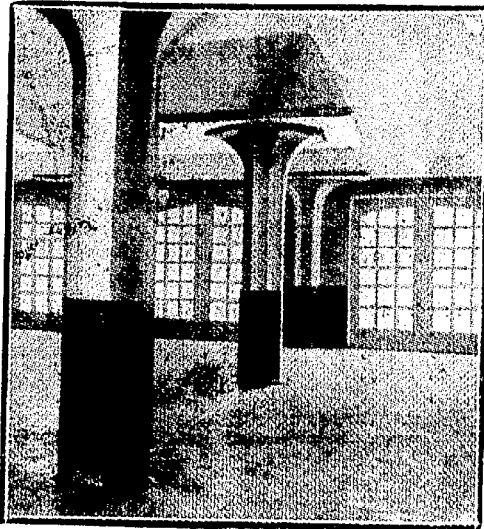
CONSTRUCTIONS IN REINFORCED CONCRETE Speciality - FLAT SLAB SYSTEM. Ford Building - São Paulo - built by us is the first example of this system in Brazil.
