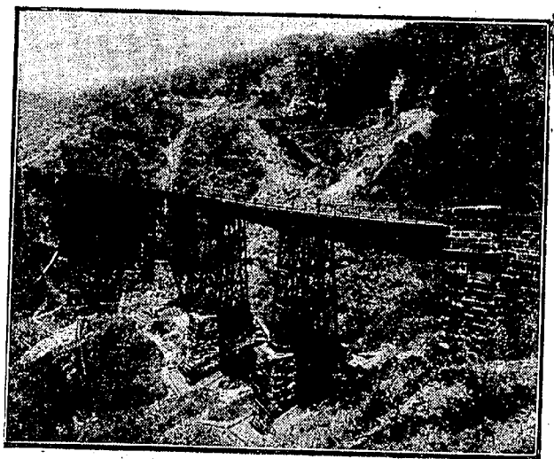
The Grota Viaducts on the Inclined Planes, showing Old and New Foundations.
