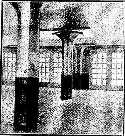
CONSTRUCTIONS IN REINFORCED CONCRETE Specialty - FLAT SLAB SYSTEM. Ford Building - São Paulo - built by us is the first example of this system in Brazil.
