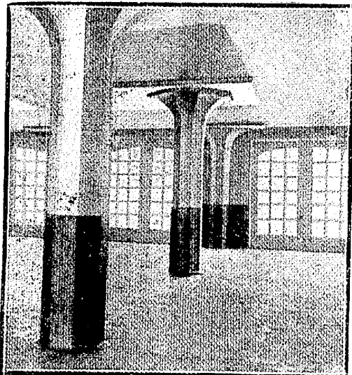
CONSTRUCTIONS IN REINFORCED CONCRETE Specialty - FLAT SLAB SYSTEM. Ford Building - São Paulo - built by us is the first example of this system in Brazil.
