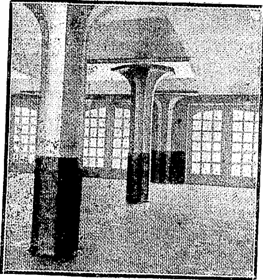
CONSTRUCTIONS IN REINFORCED CONCRETE Speciality - FLAT SLAB SYSTEM. Ford Building - São Paulo - built by us is the first example of this system in Brazil.
