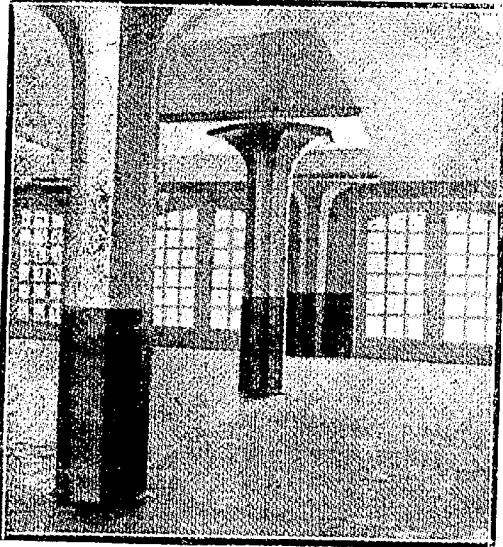
CONSTRUCTIONS IN REINFORCED CONCRETE Specialty - FLAT SLAB SYSTEM. Ford Building - São Paulo - built by us is the first example of this system in Brazil.
