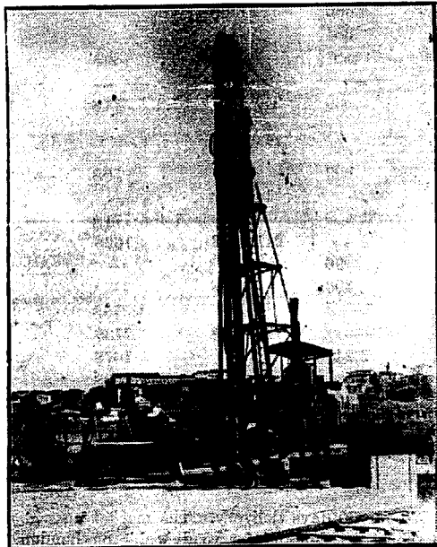
DRIVING CONCRETE PILES PORTLANDS, RIO DE JANEIRO. 2 ton Steam pile hammer.
