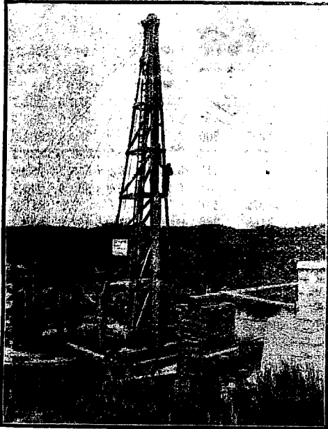
FALSE WORK FOR STEEL ERECTION.
