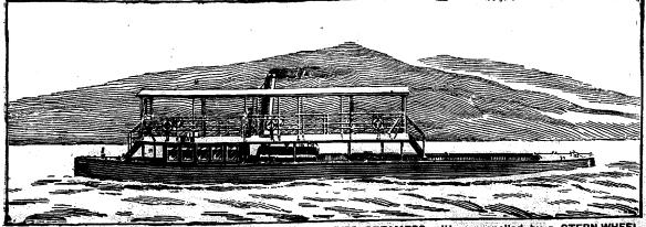
YARROW'S make a speciality of SHALLOW-DRAUGHT RIVER STEAMERS, either propelled by a STERN-WHEEL or by SCREWS WORKING IN TUNNELS, fitted with YARROW'S PATENT HINGED FLAP, by which means a considerable increase in speed is obtained without increase of cost. Vessels can be delivered whole, in pieces, or in floatable sections arranged so that they may be readily united while afloat.
