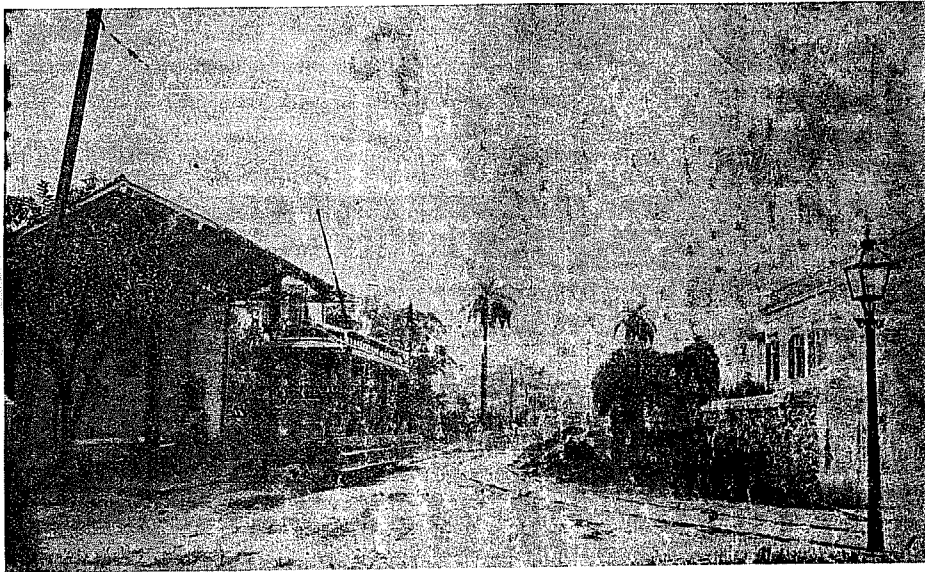
JUNCTION AT THE RUA CONDE BOMFIM
