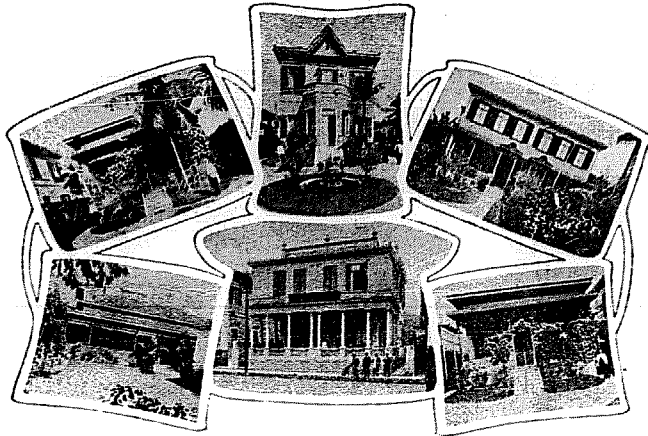
(Buildings composing the Hotel)
