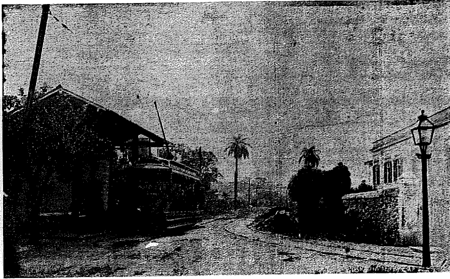
JUNCTION AT THE RUA CONDE BOMFIM
